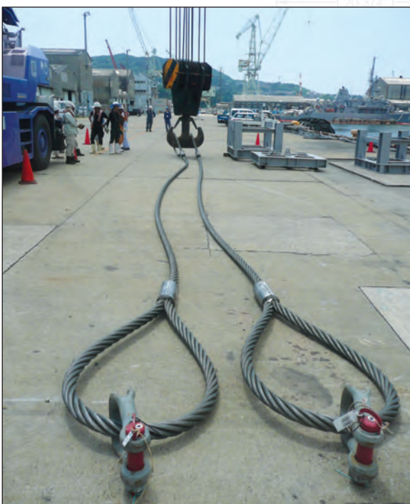
Rigging preparations for 150kip load test for shipboard system
